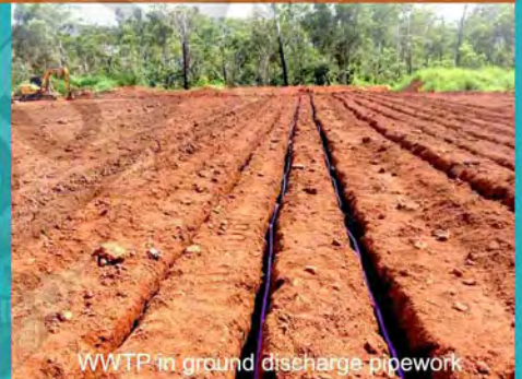
Pipework from tank
